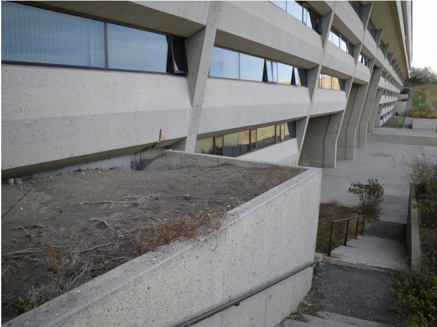
East Retaining Walls, Planters, Stairs and Sidewalks – View of South Segment North of Level 6 Patio
