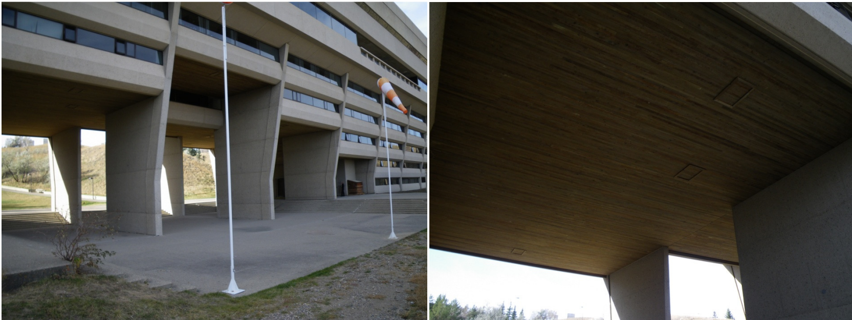
Breezeway Soffit – View from Breezeway
