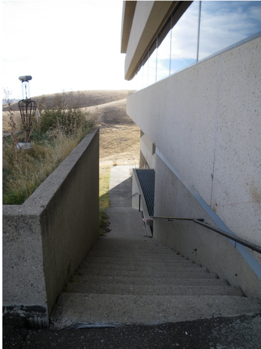
East Retaining Walls, Planters, Stairs and Sidewalks – View of South Segment South of Level 6 Patio
