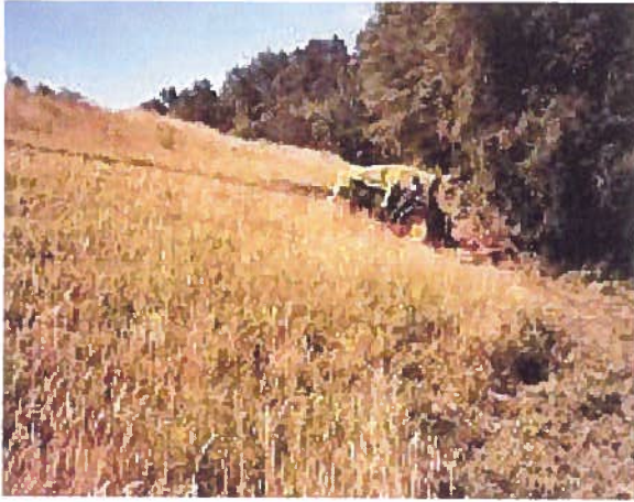
Grass on dams requires regular mowing.
