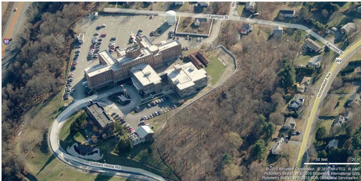
Aerial View of Soldiers' Home in Holyoke
