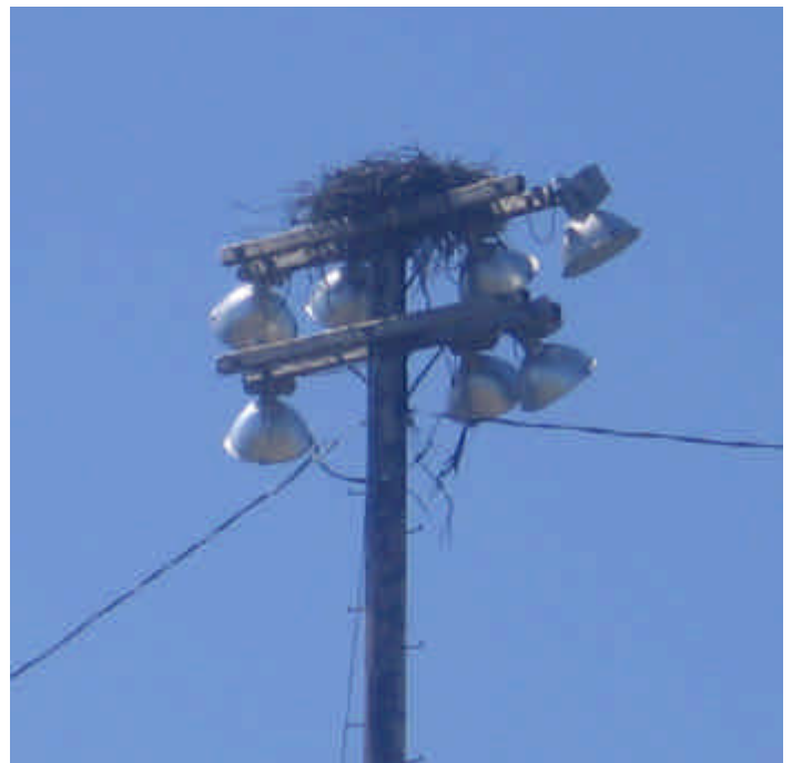
Figure 6 - D Birds nest is sitting on top of the top light bar.
