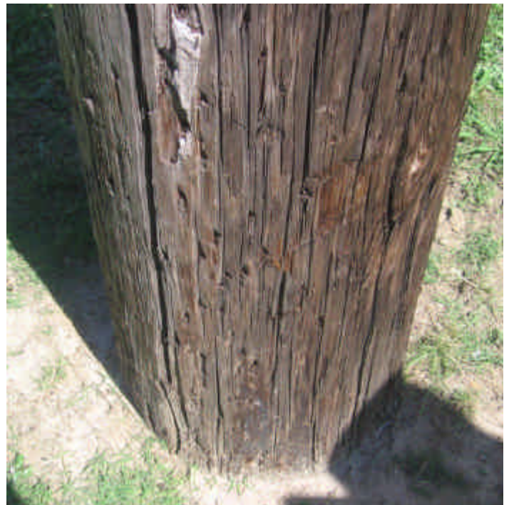
Figure 7 - D Vertical checks. Moisture and incising treatment is indicated by the small holes.
