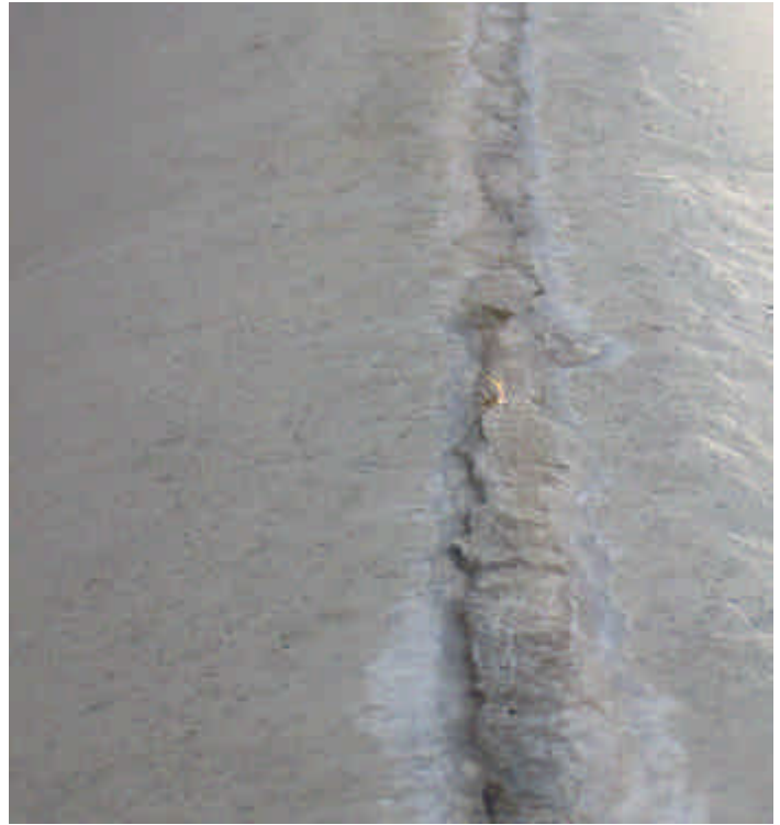
Figure 7 - B Repair material on vertical crack at formwork edge.
