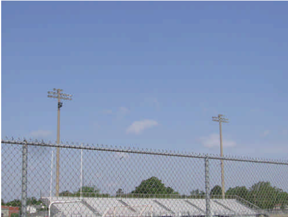
Figure 1 - A View of typical High-Level (Pole Type) light poles
