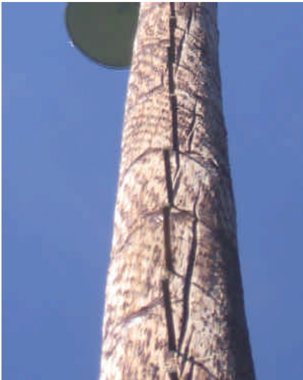
Figure 8 - C Vertical checks near the pole hand holds.
