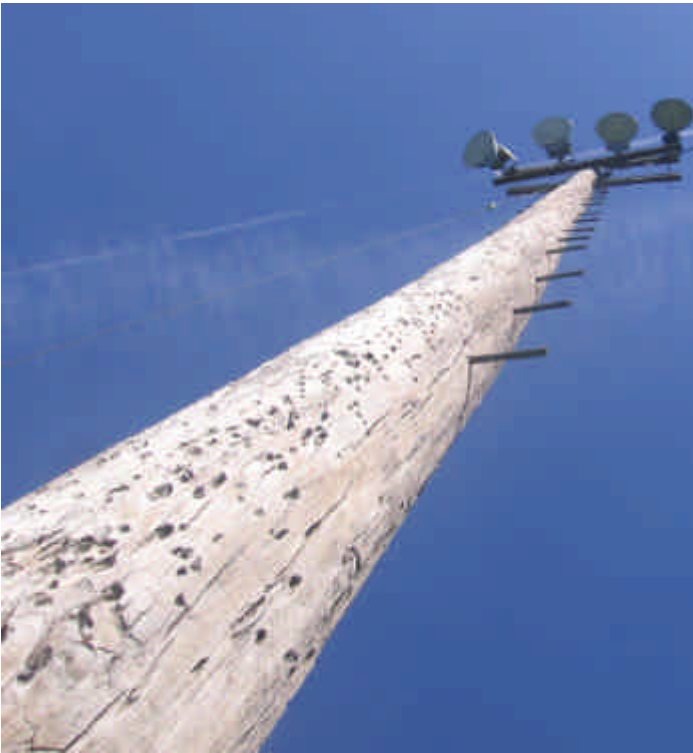
Figure 9 - A Small holes on upper half of pole not caused by incising treatment.
