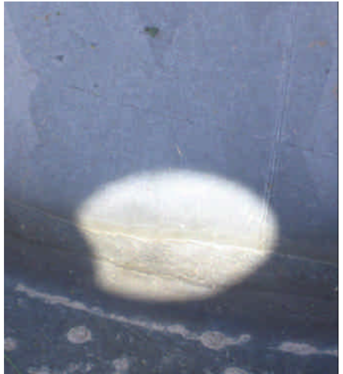
Figure 2 - B No cracks at the welded connection were visually observed.
