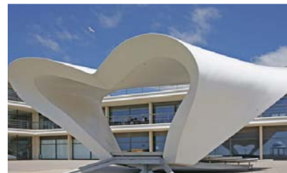
Bandstand, Niall McLaughlin Architects
