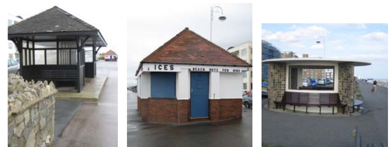
Above, existing seafront structures to be replaced
