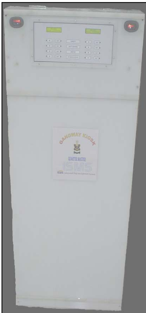
Front View of Gangway Kiosk
