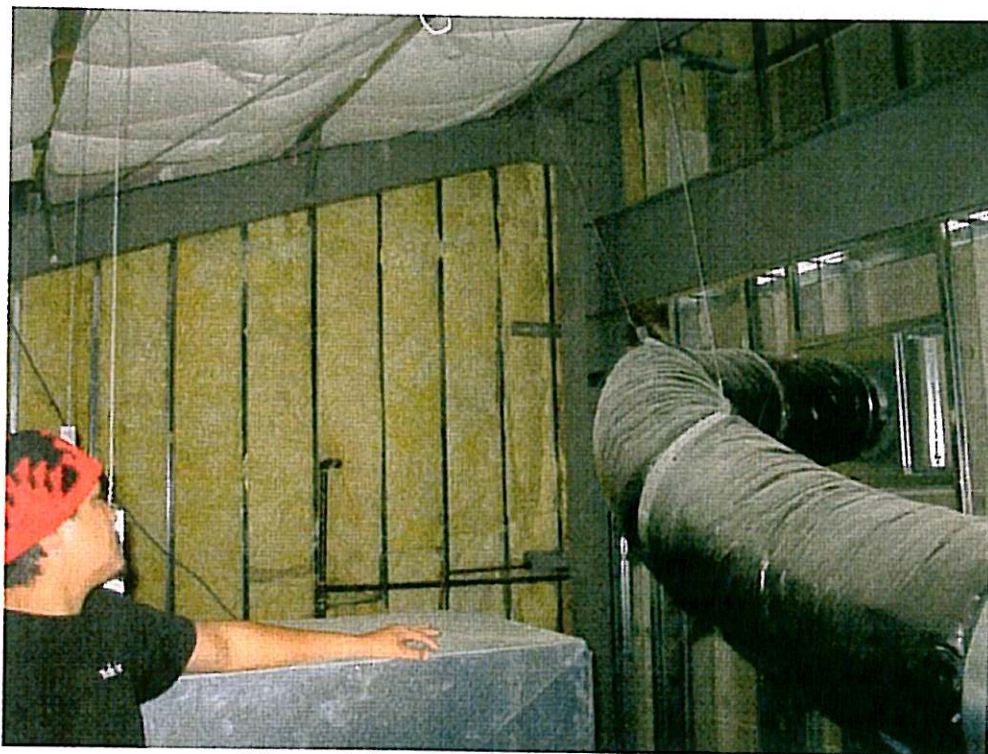
Figure 3. Insulated attic above kitchen
