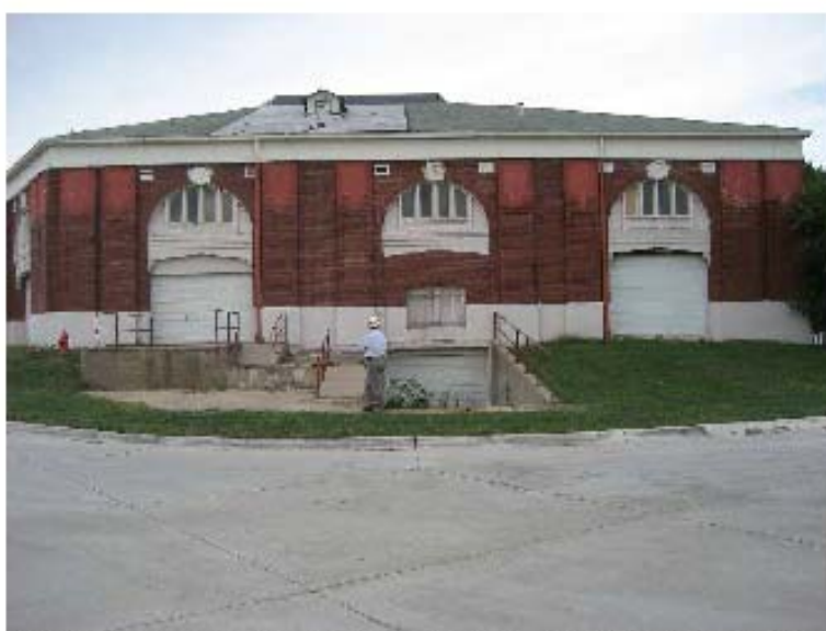
Figure 10 —Photo of east façade. Note concrete ramp and retaining walls leading to lower level. Photo - D.Worth and S. Kelley Sept 2009
