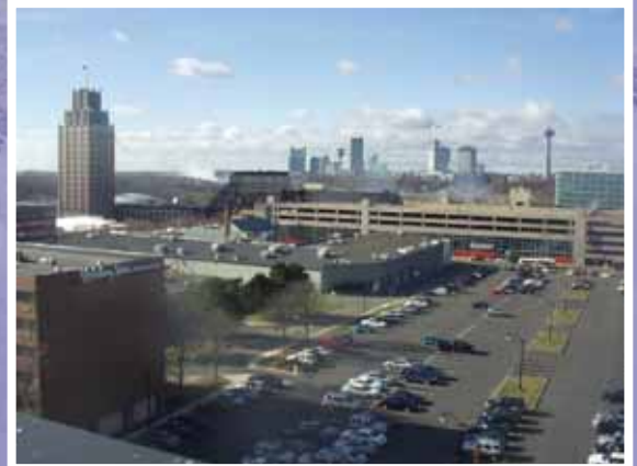
View of the project site to the southwest, showing Holiday Inn (Crowne Plaza) and United Office Building sites.
