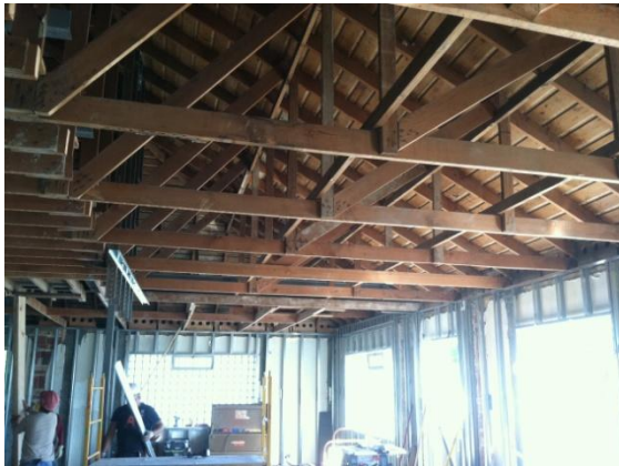
New Summit County Library, Coalville, Utah Under Construction – August 2011 View of rafters/open ceiling work planned for facility
