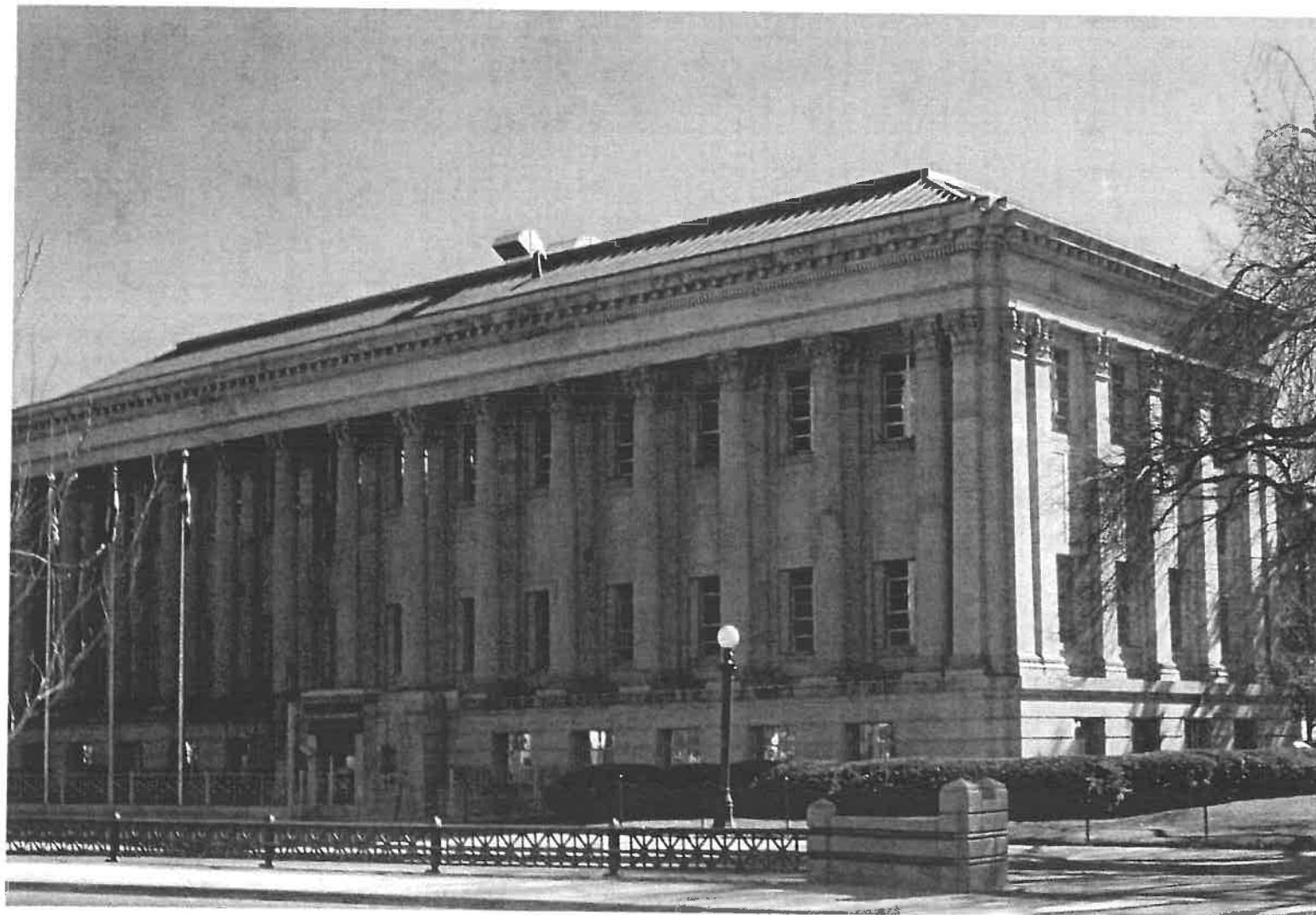
Left: North entrance showing building entrance at lower level, prominent mechanical vents in lieu of skylight, mismatching stone covering frieze inscription and original window openings, ca. August 2009
