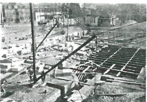
Historic construction foundation 3
