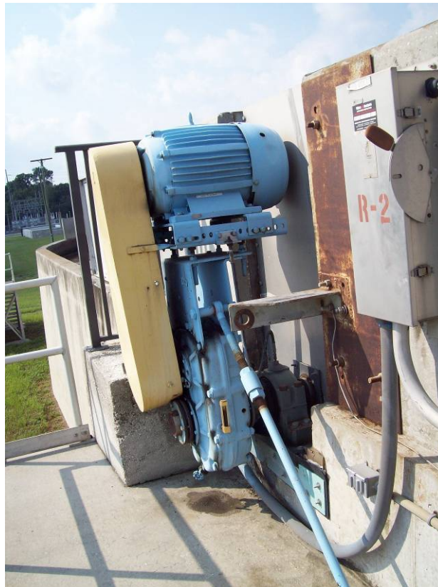
Figure 2.5. Drive mechanism for Brush Aerators
