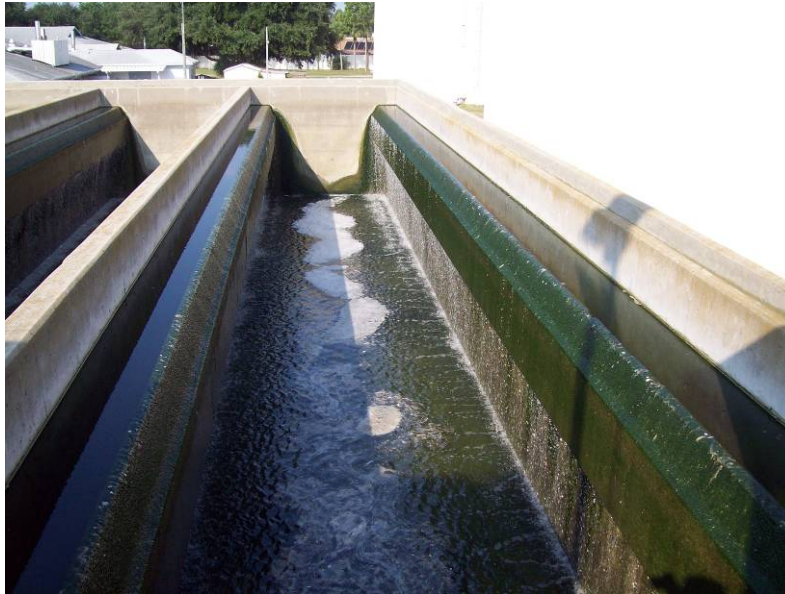
Figure 2.4. Deep Bed Filters
