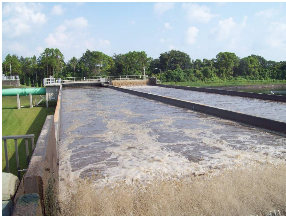
Figure 2.6. Oxidation Ditches
