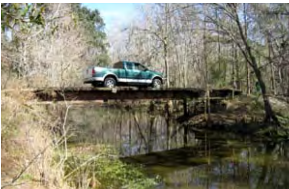
Steel bridge over Prairie Creek
