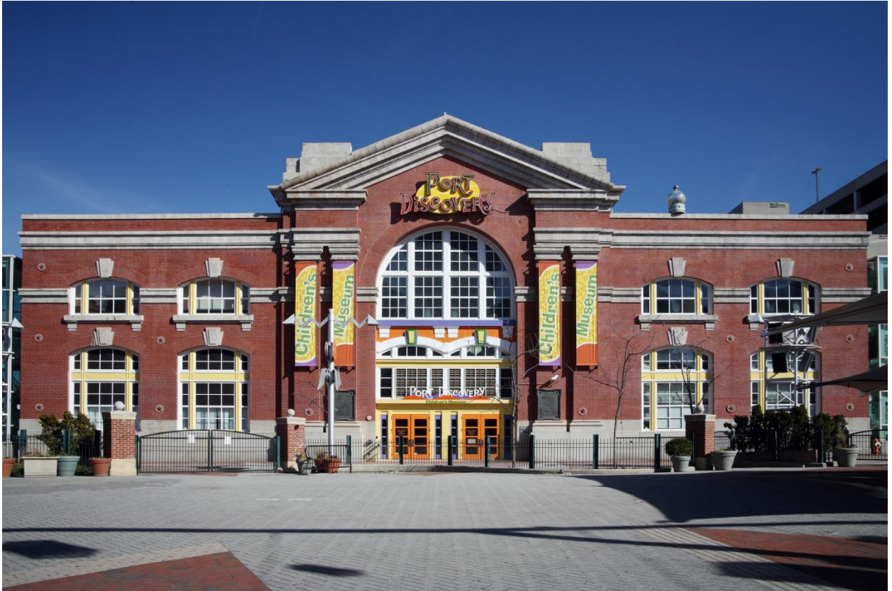
Port Discovery Children's Museum today. Opened in December 1998, the 80,000 square foot facility served as the anchor for the redevelopment efforts of the City in the eastern basin of the Inner Harbor.
