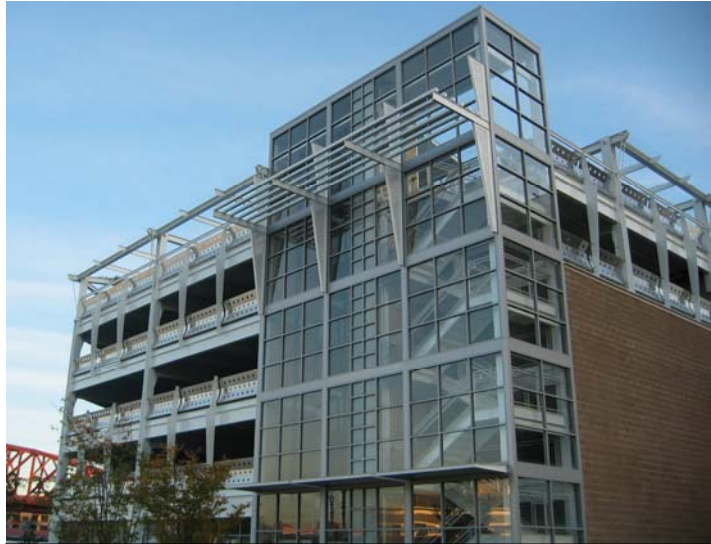
Photo: Station Place Garage
