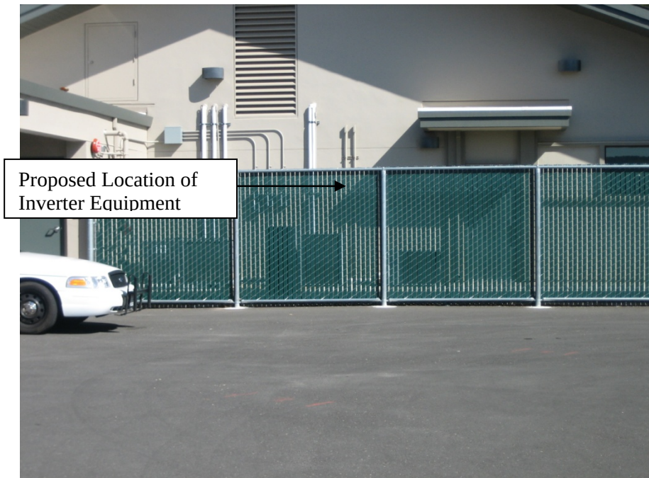
Photo 4 – Proposed Location of Inverter Equipment
