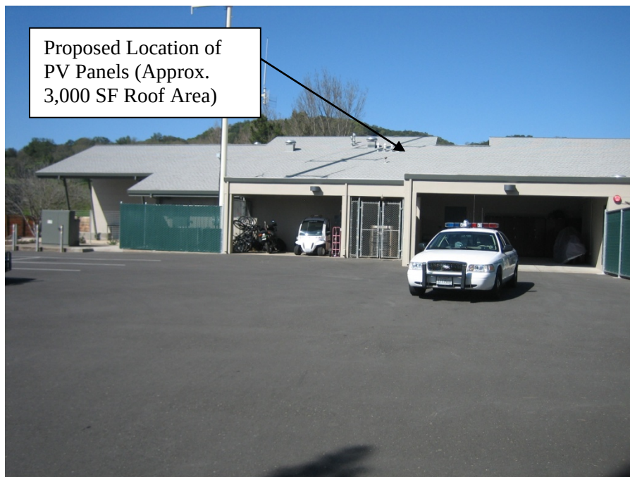
Photo 2 – Proposed Location of PV Panels on Roof
