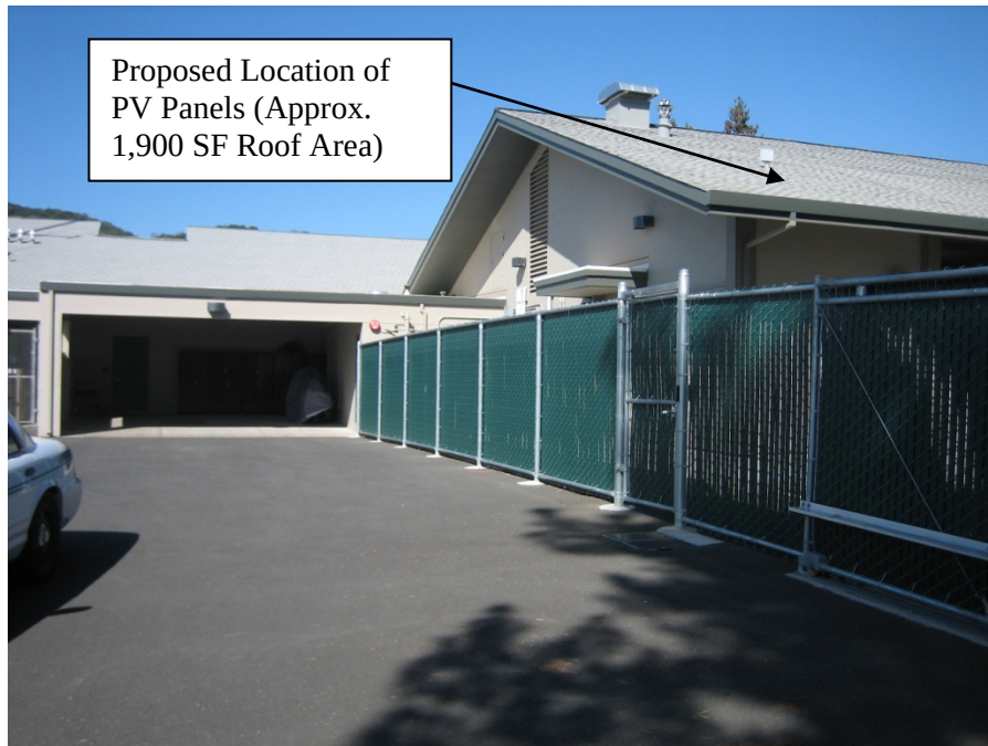
Photo 1 – Proposed Location of PV Panels on Roof
