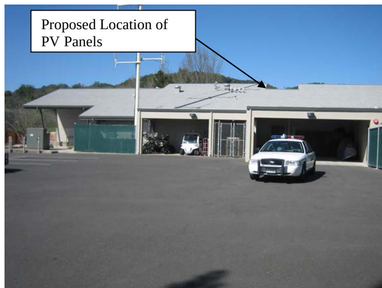
Image 8 - Police Station PV Panel Location
