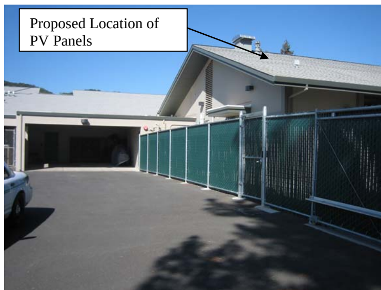
Image 7 - Police Station PV Panel Location
