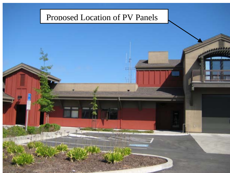
Image 5 - Fire Station Roofing System
