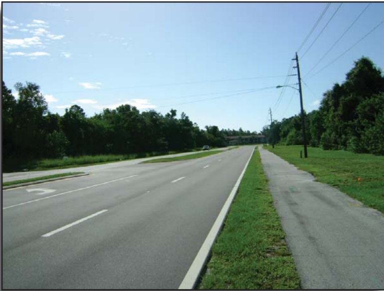
Photo 1 Looking south on Troutman Blvd at the beginning of the project limits.
