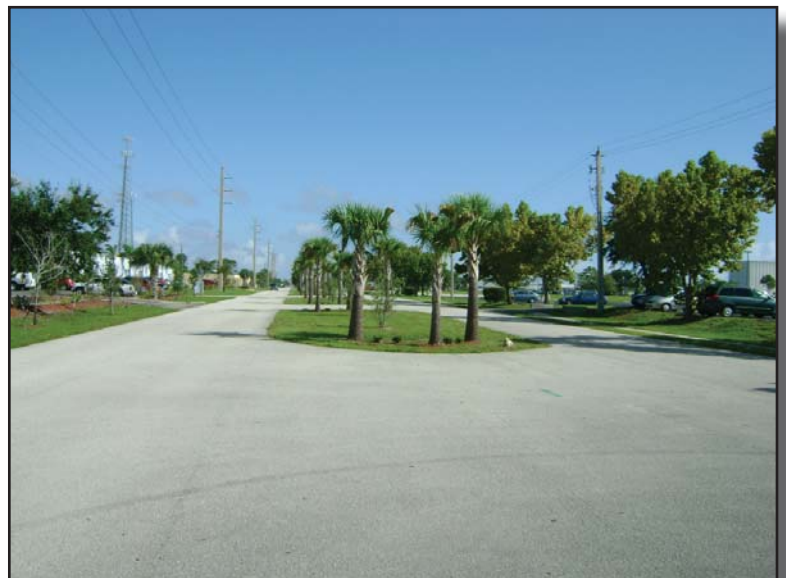
Photo 6 Looking north at Clearmont Street, just north of proposed tie-in.
