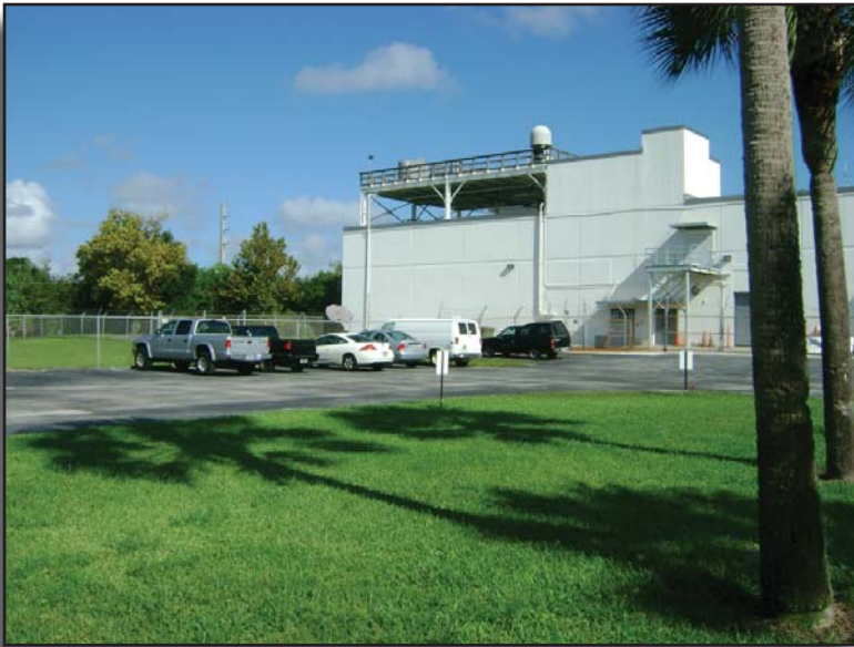
Photo 4 Proposed alignment will impact existing fence.
