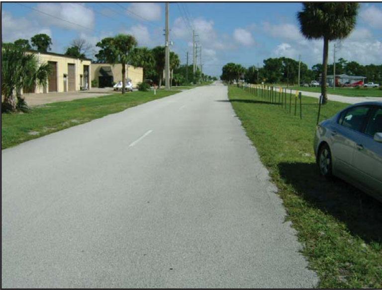
Photo 13 Existing pavement in fair to good condition south of Franklin Drive on Clearmont Street.
