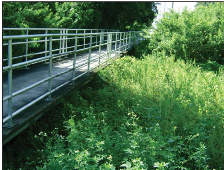
Photo 8 Existing creek just south of our project limits.
