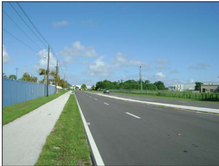
Photo 2 Looking north on Troutman Blvd at the beginning of the project limits.
