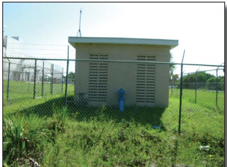
Photo 9 Location of existing utility just south of proposed alignment.
