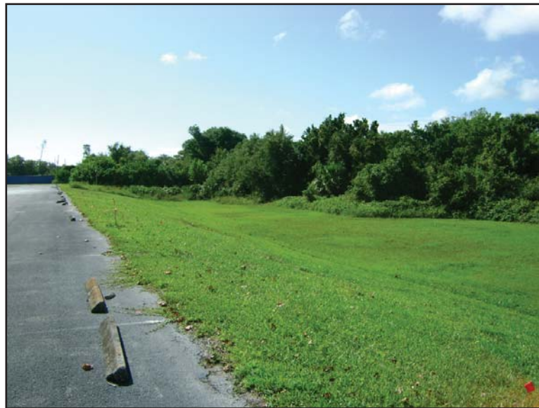
Photo 11 Existing stormwater for Harris parking lot will be expanded for stormwater treatment.
