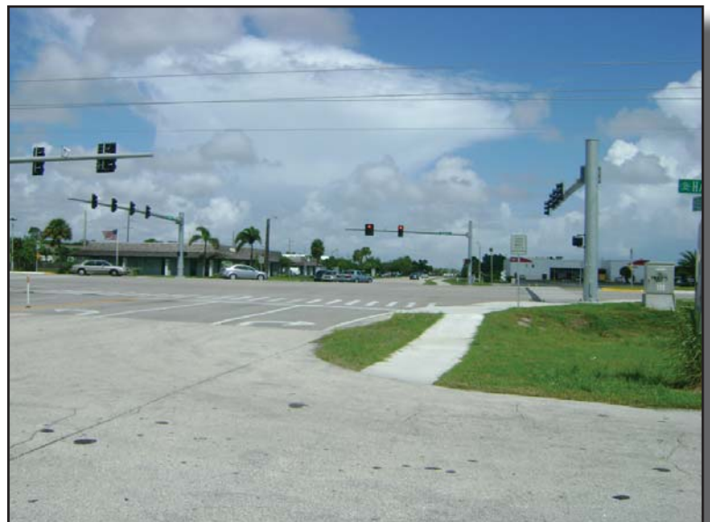
Photo 15 End of project study area at Palm Bay Road and Clearmont Street.
