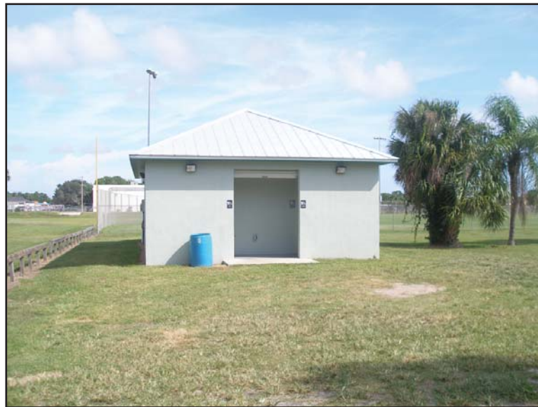
Photo 5 Existing restroom facility adjacent to softball fields.
