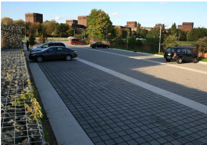
Impervious pavement in parking lot
