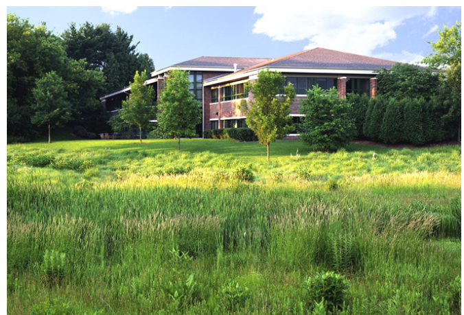
Natural appearing stormwater management system
