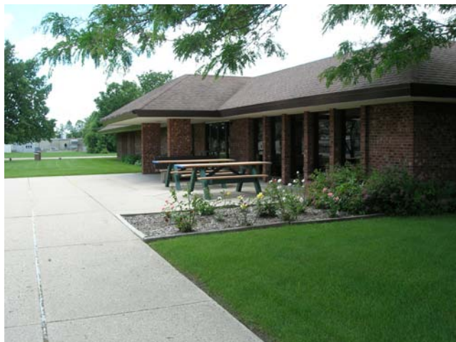
Existing campus building
