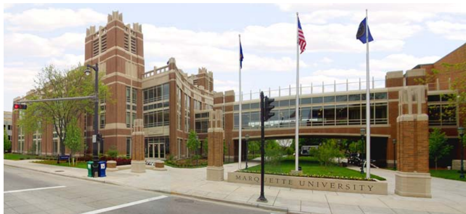
Major gateway integrated with campus architecture
