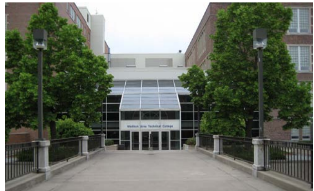
Existing building entrance from Wisconsin Avenue
