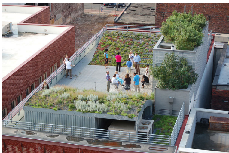
“Greenroof” retrofit to existing building
