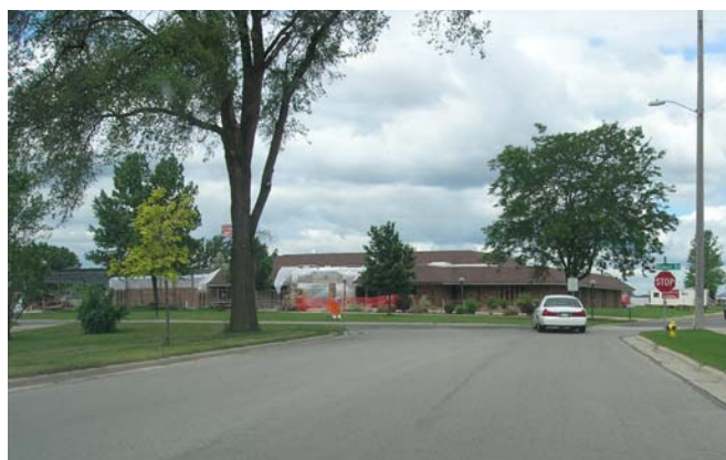
Existing campus building
