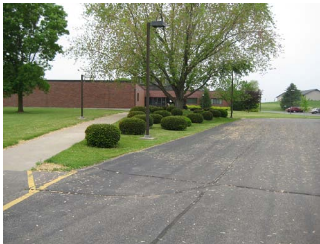
Existing campus building
