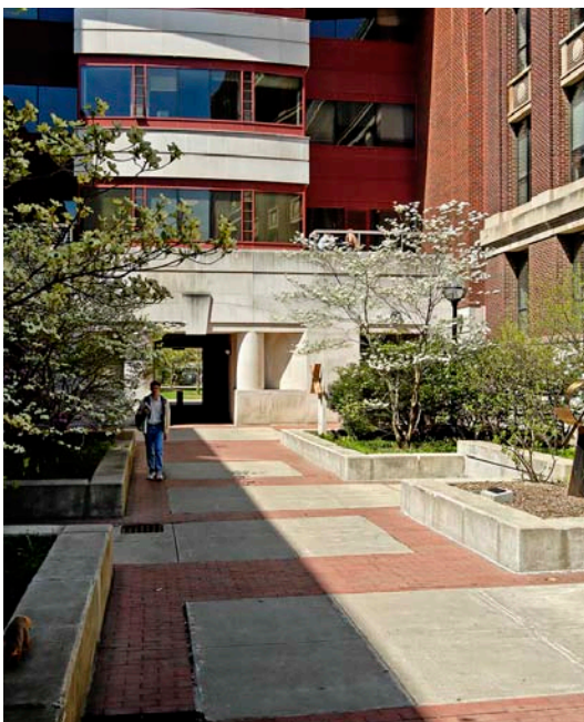
Interior courtyard with tunnel connection
