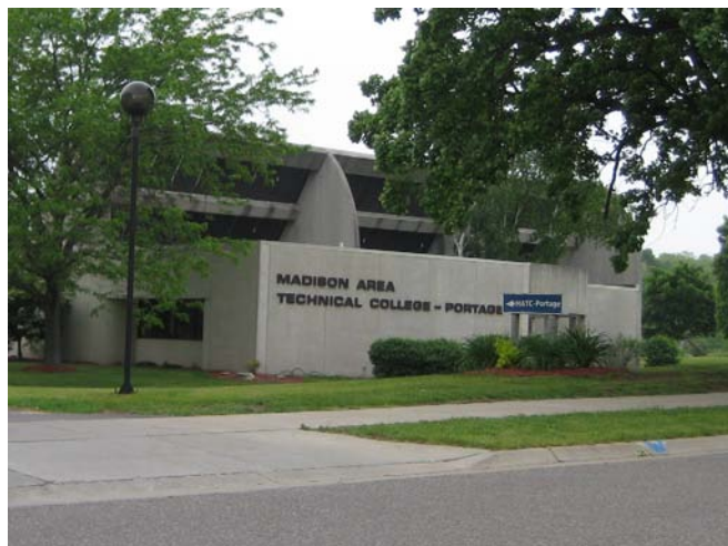
Existing campus building
