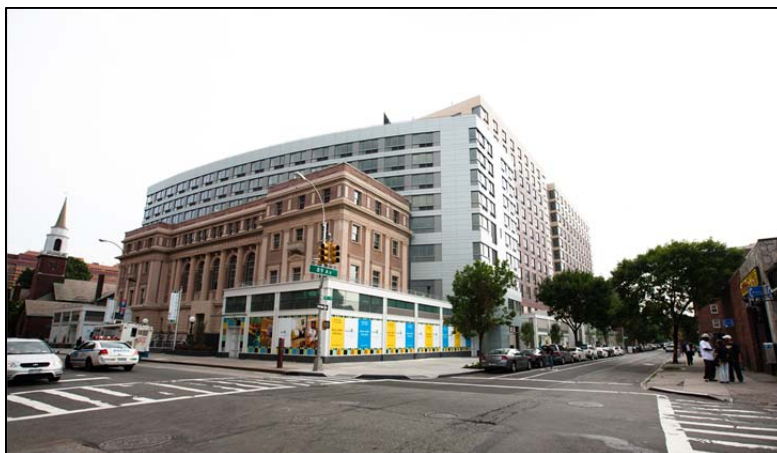
MODA project on Parsons Boulevard, downtown Jamaica
