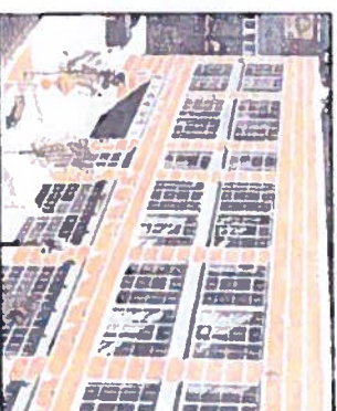
Brick and glass allow this parking structure to maintain a more sensitive relationship with its context.
