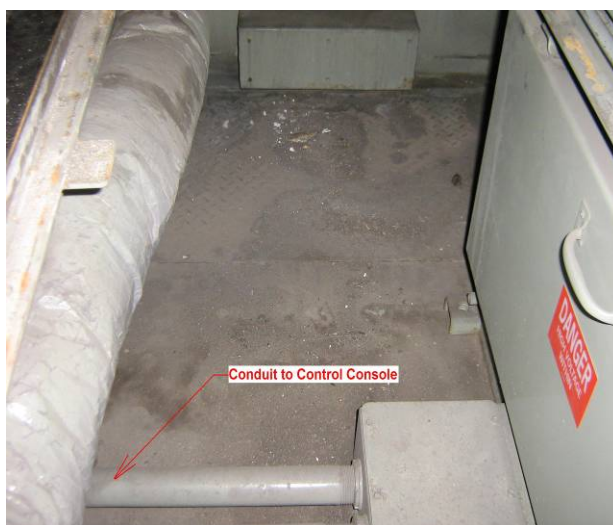
Sub Floor (Access Panel Removed)
