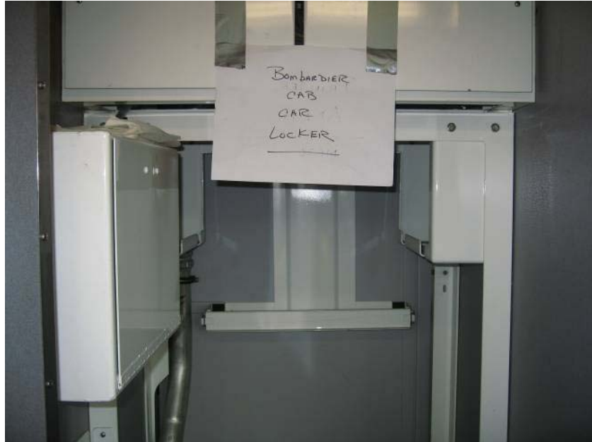
Figure 39 - Equipment Locker - Bombardier Cab Car
