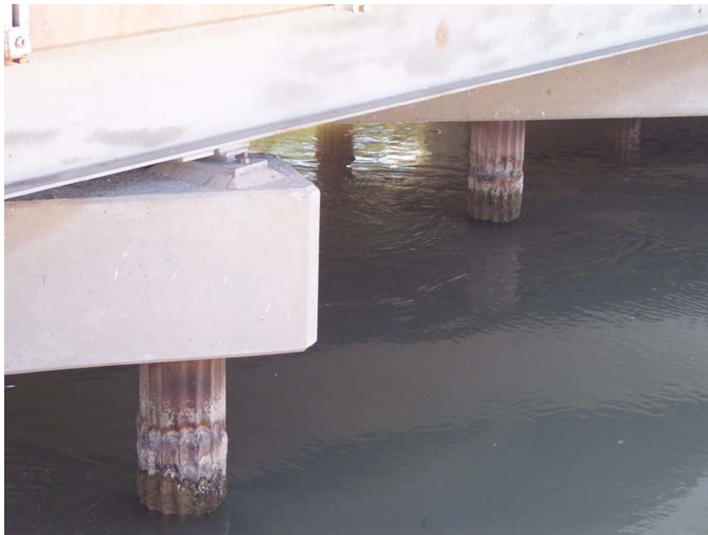
Figure 6: Bridge Pilings Facing Northwest June 19, 2008
