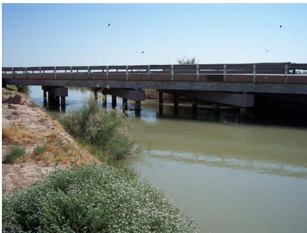
Figure 14: Bridge Facing East June 19, 2008
