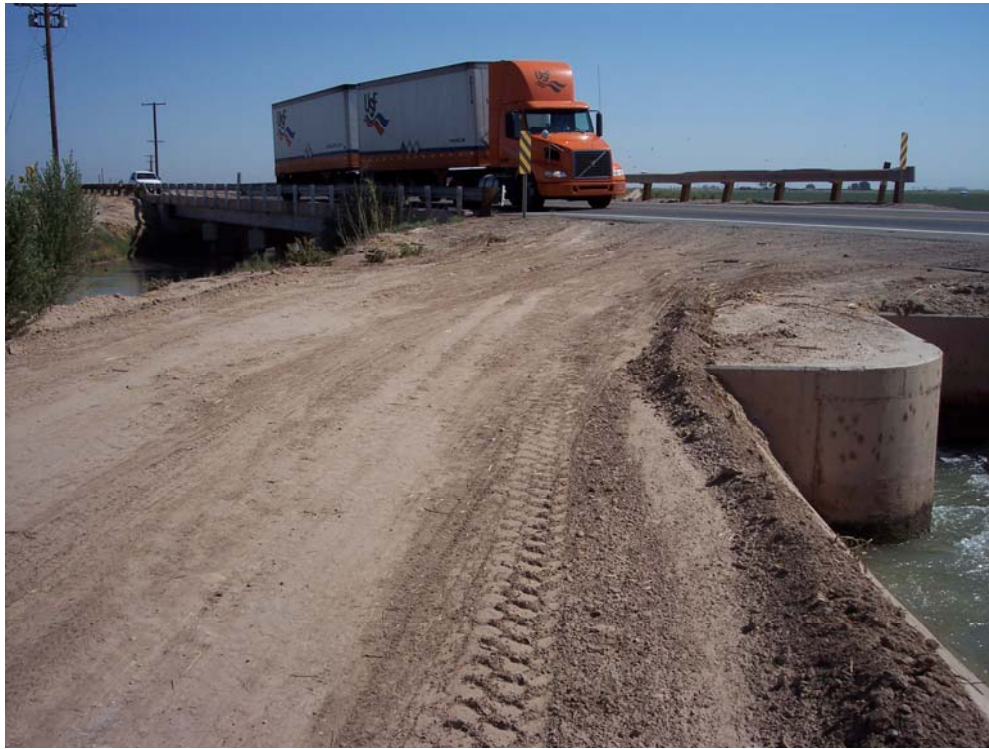
Figure 9: Westside Main and Sumac Canal Facing Northeast June 19, 2008
