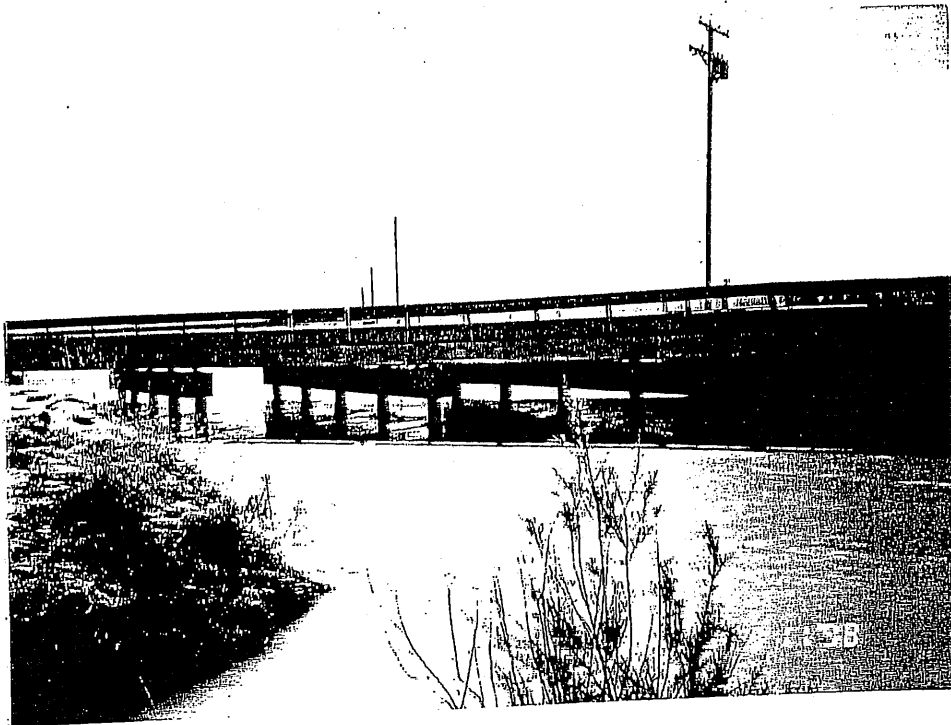
200-6-15 Main Canal and east side of bridge
