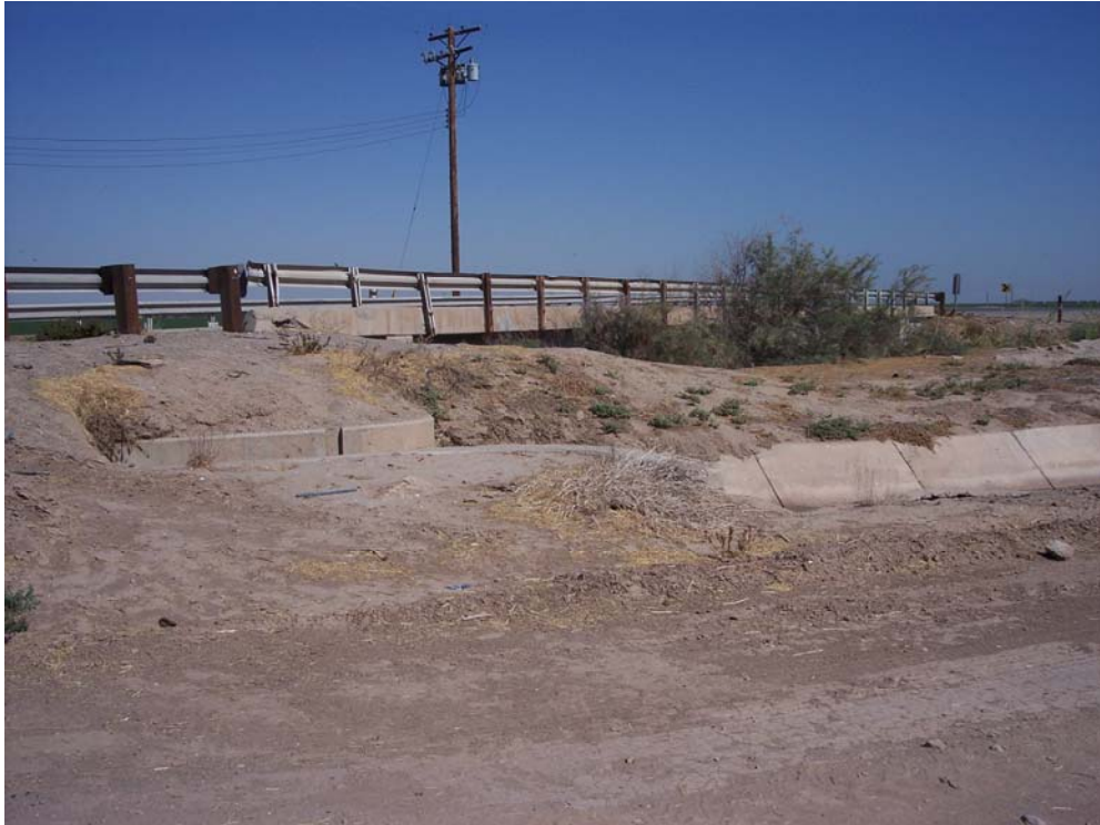
Figure 3: Sumac Canal Headgate on East Side June 19, 2008
