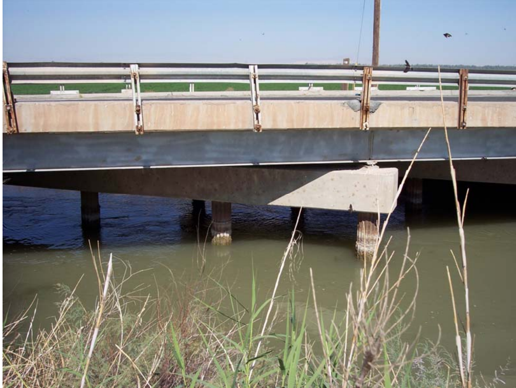
Figure 5: Bridge Pilings Facing Northwest June 19, 2008
