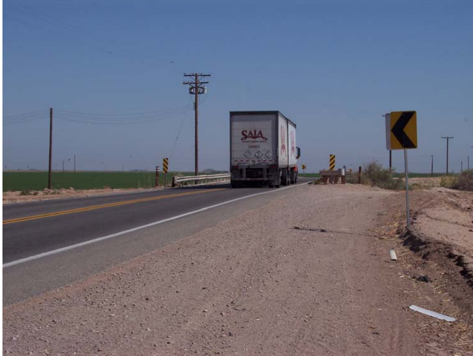
Figure 1: Northbound Approach Facing Northwest June 19, 2008
