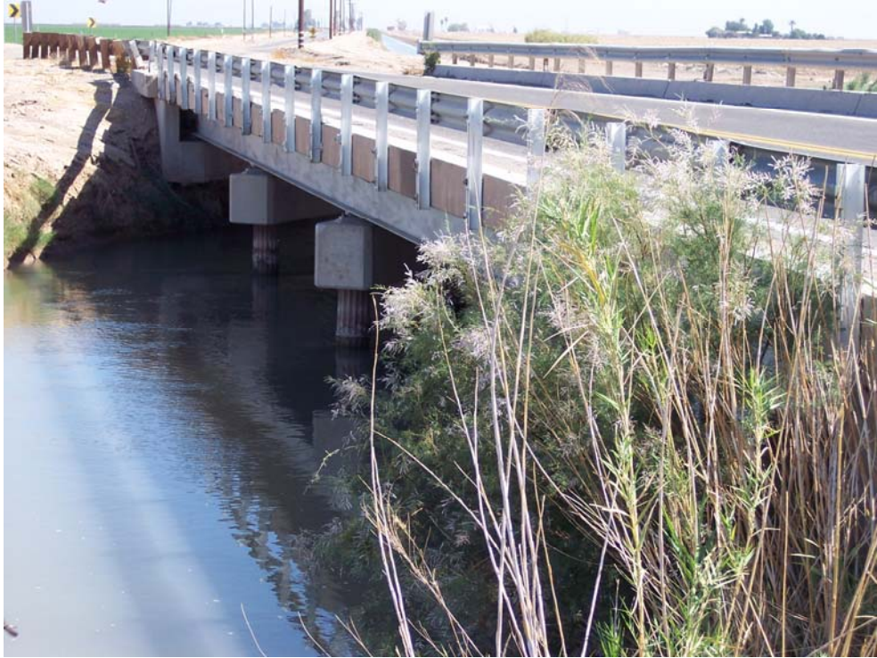
Figure 7: Bridge Pilings Facing Northeast June 19, 2008
