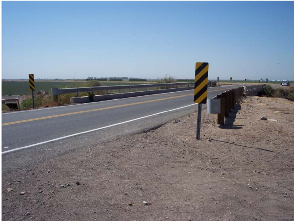
Figure 11: Southbound Approach Facing Southeast June 19, 2008
