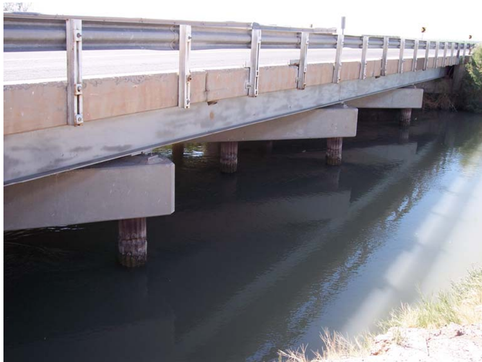
Figure 8: Bridge Pilings Facing Southeast June 19, 2008
