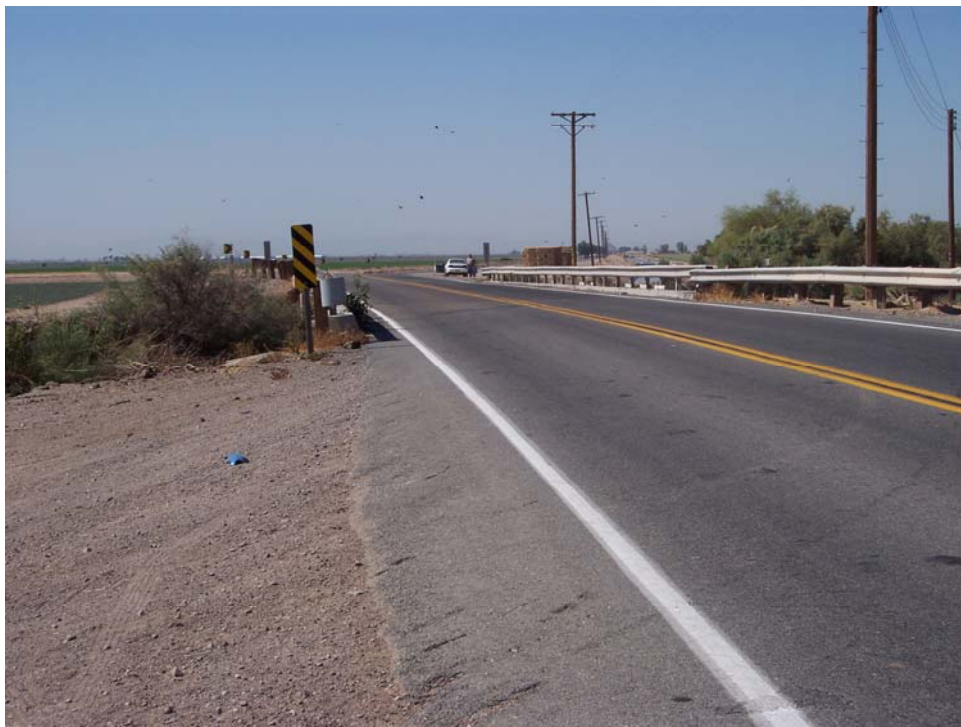
Figure 12: Southbound Approach Facing Southwest June 19, 2008
