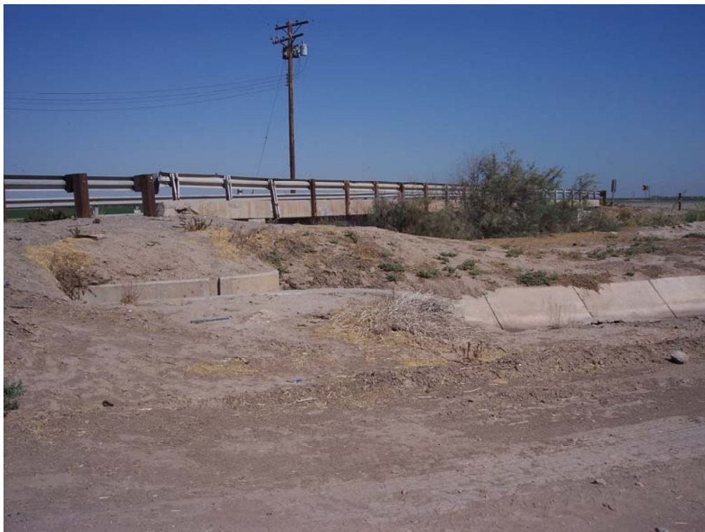
Figure 4: Overlooking Sumac Canal Facing Northwest June 19, 2008
