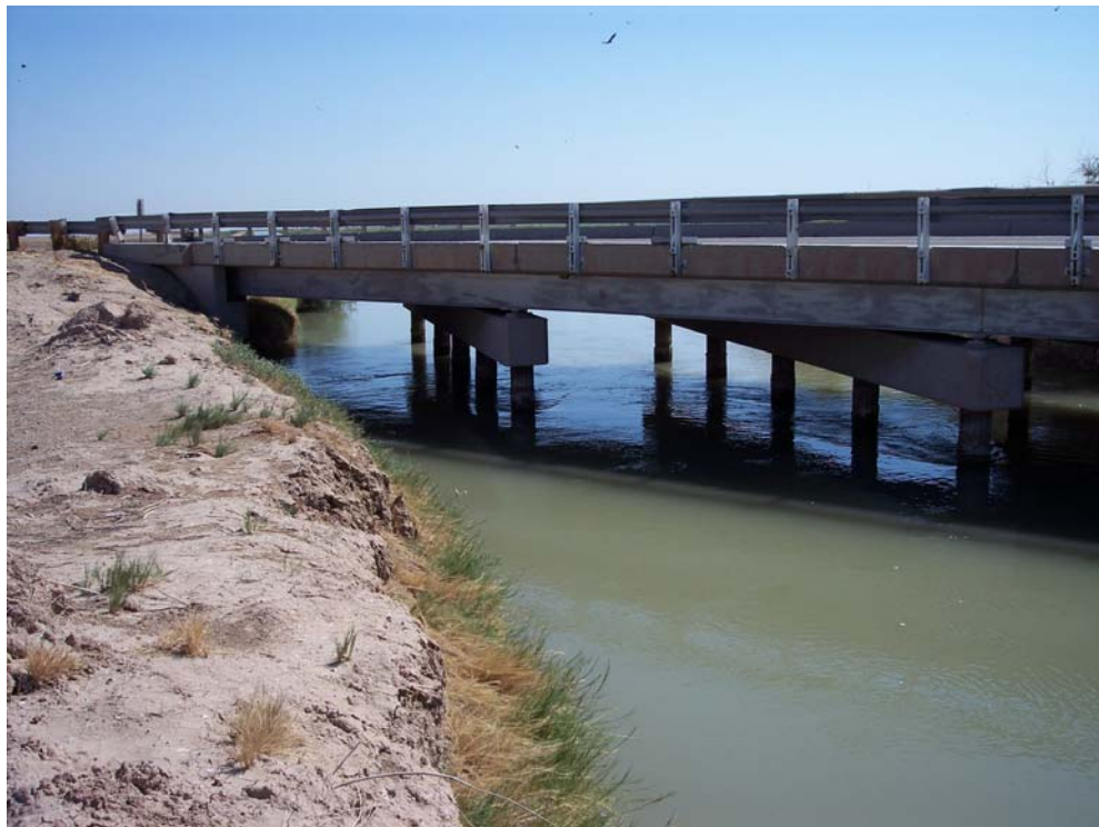
Figure 10: Northern End of Bridge Facing East June 19, 2008
