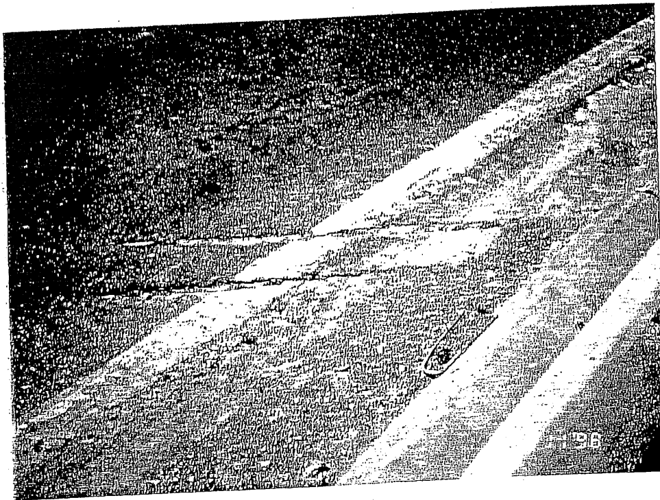
200-6-19 South abutment AC overlay cracks
