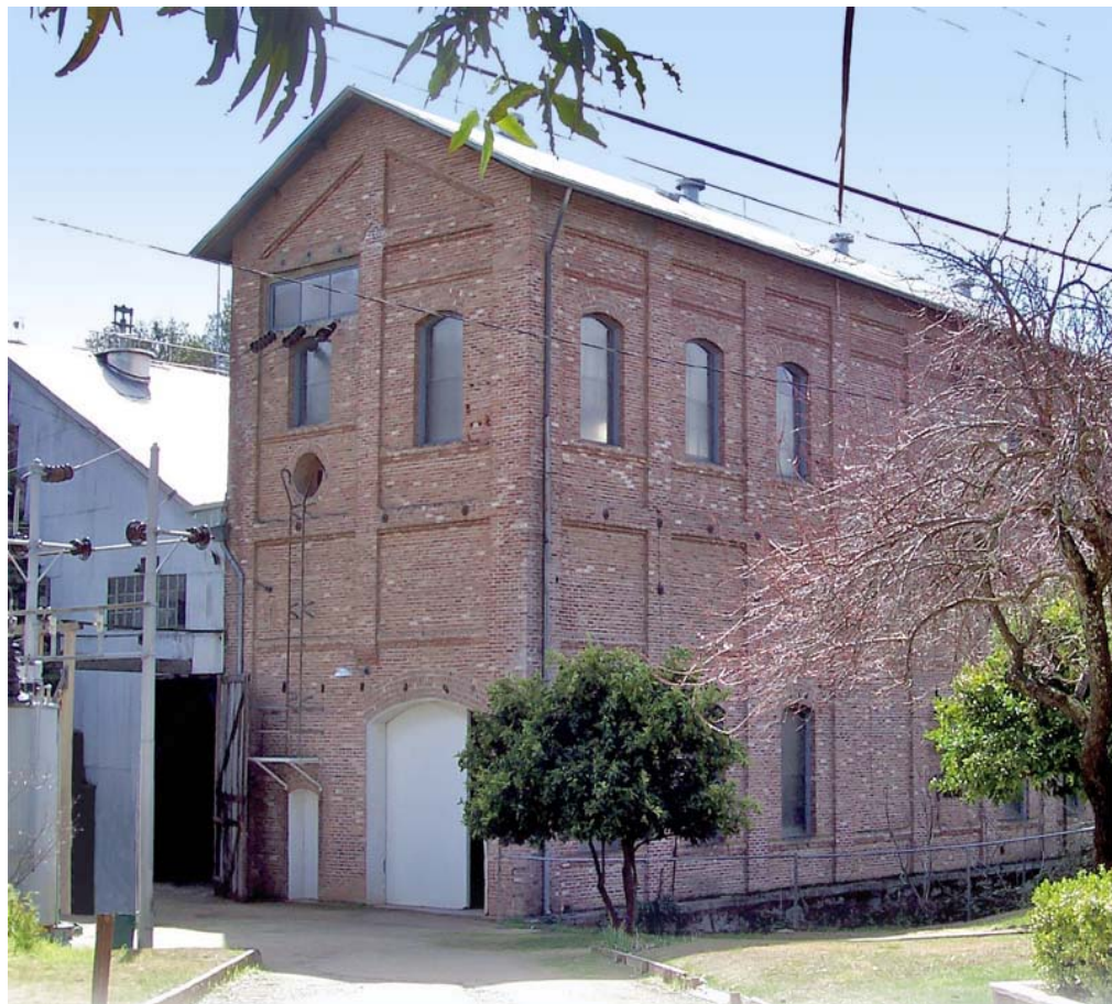
Figure 2 - Restoration of the main generator building at the Folsom Powerhouse SHP occurred in 2006.
