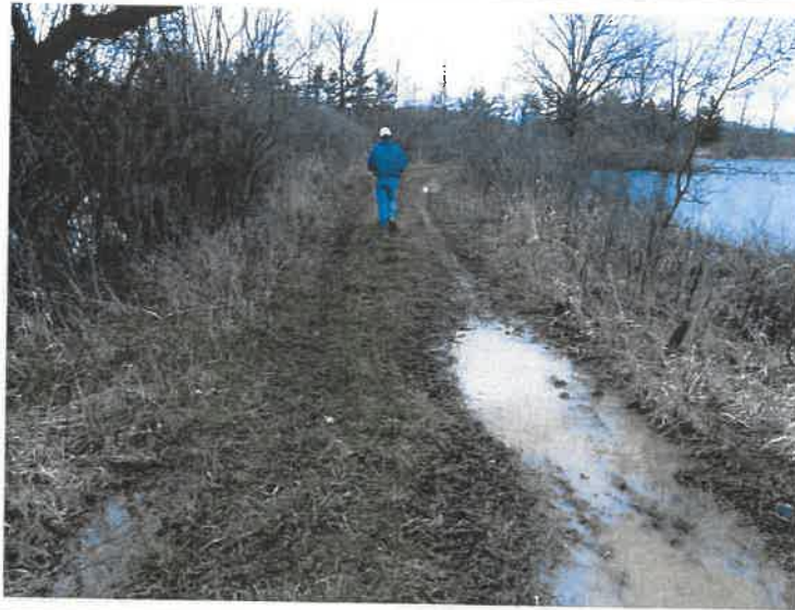
4. A view of the crest of the saddle dam.
