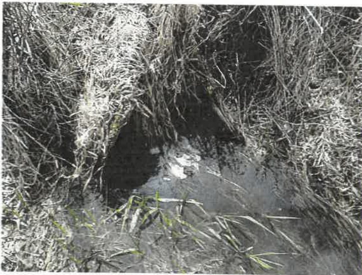
12. A view of the principal spillway outlet.
