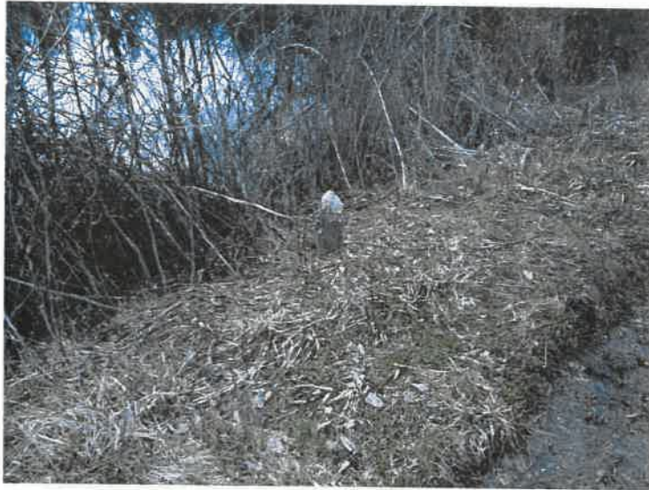
7. A view of the downstream slope of the saddle dam.
