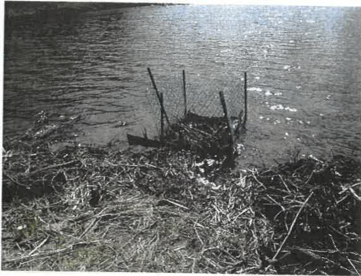
10. A view of the principal spillway riser and trashrack
