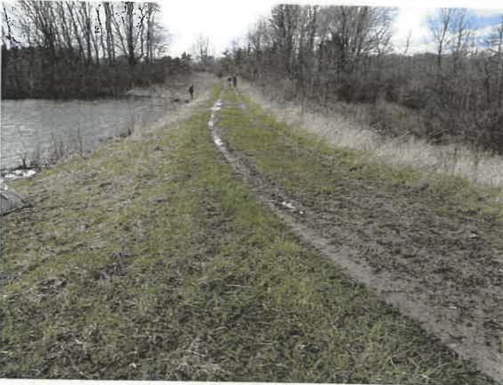
5. A view of the crest of the main dam.
