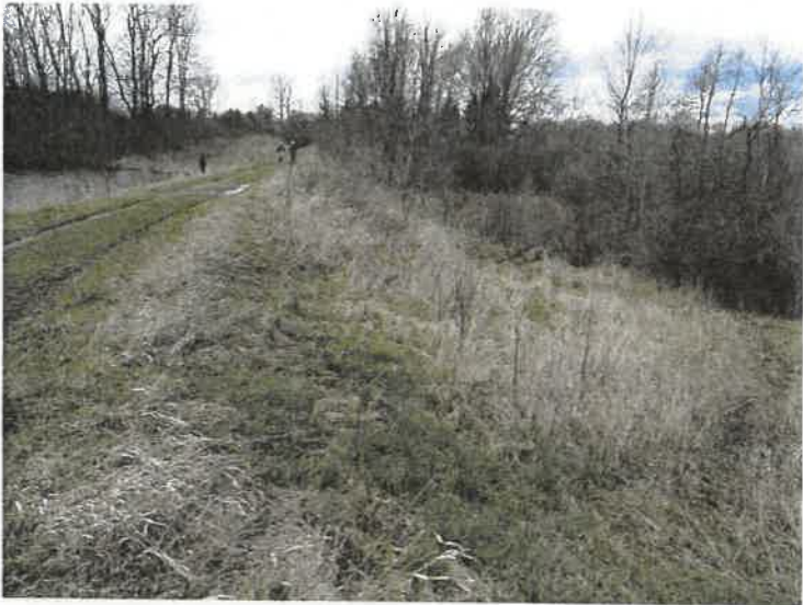
8. A view of the downstream slope of the main dam.
