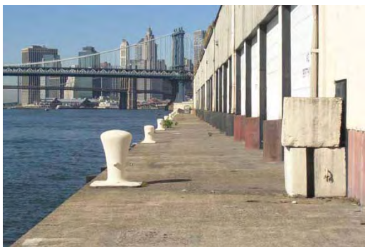
Overall view of Pier 42 apron, looking south.
