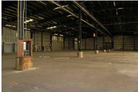
Overall view of the interior of the Pier Shed.
