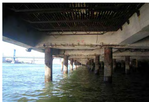
Pier 42 substructure, looking south.
