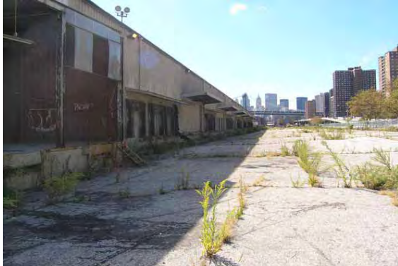
Overall view of the Site from the open area, looking south.
