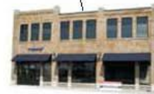
300 Ellsworth Administrative Offices
