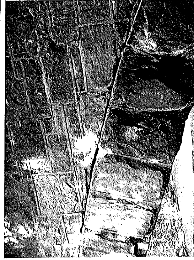
Photo # 16: Span 1, south elevation, east end: Deteriorated mortar between the arch ring stones and the spandrel wall.
