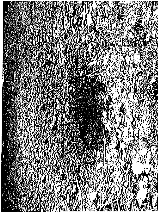
Photo # 25: Scour hole at the southeast channel embankment.
