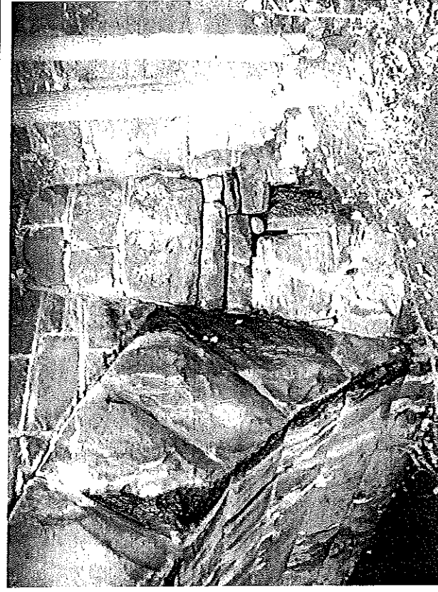
Photo # 18: Span 1, southeast corner: Architectural stone treatment at the corner of the span has deteriorated mortar/voids between the stones. Also note the leakage through the arch ring.
