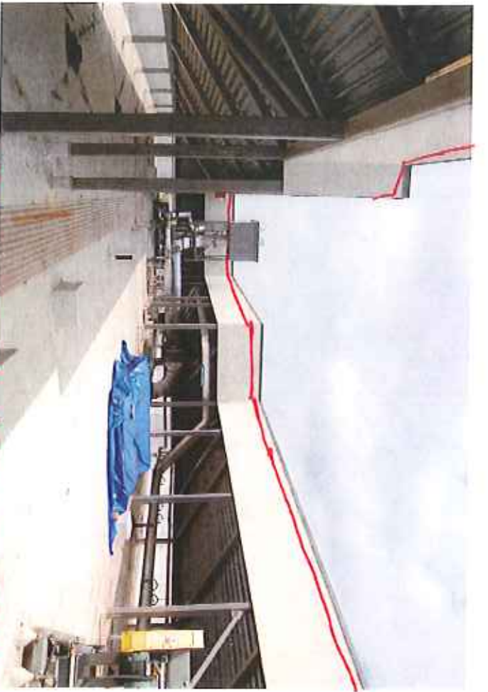
ATTACH NETTING ALONG HIGH PARAPET
