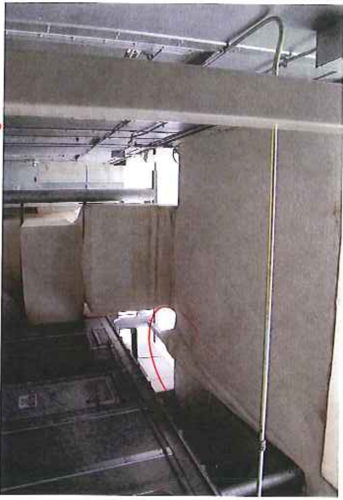
REPAIR DUCT DAMAGED BY PILEDRIVERS
