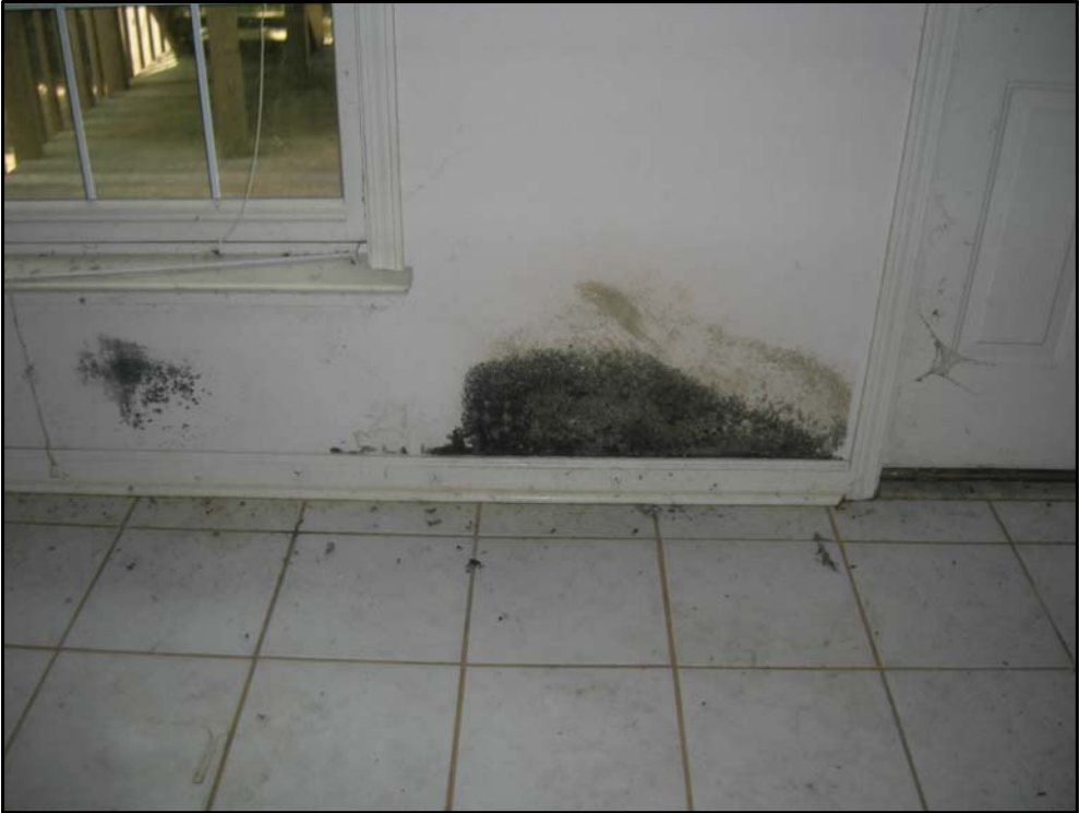
1625 REYNOLDS MILL DRIVE BASEMENT
