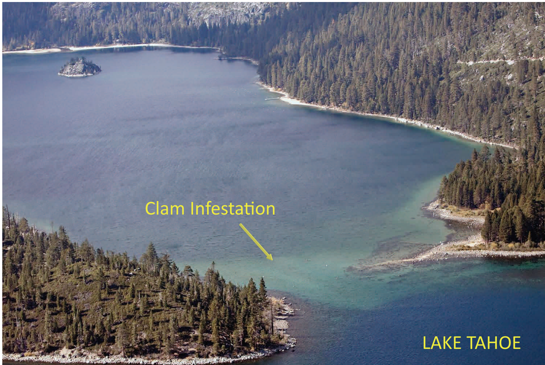
Photograph of Project Location
