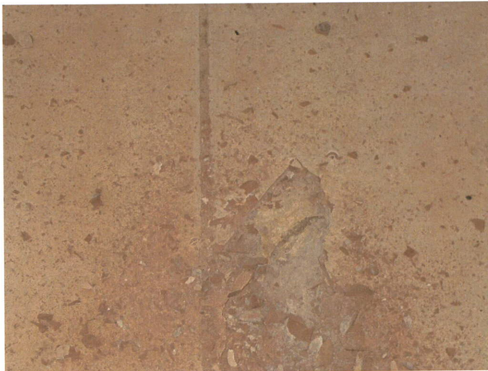
Photo 4: Typical ACM tan VFT under ceramic in water heater areas
