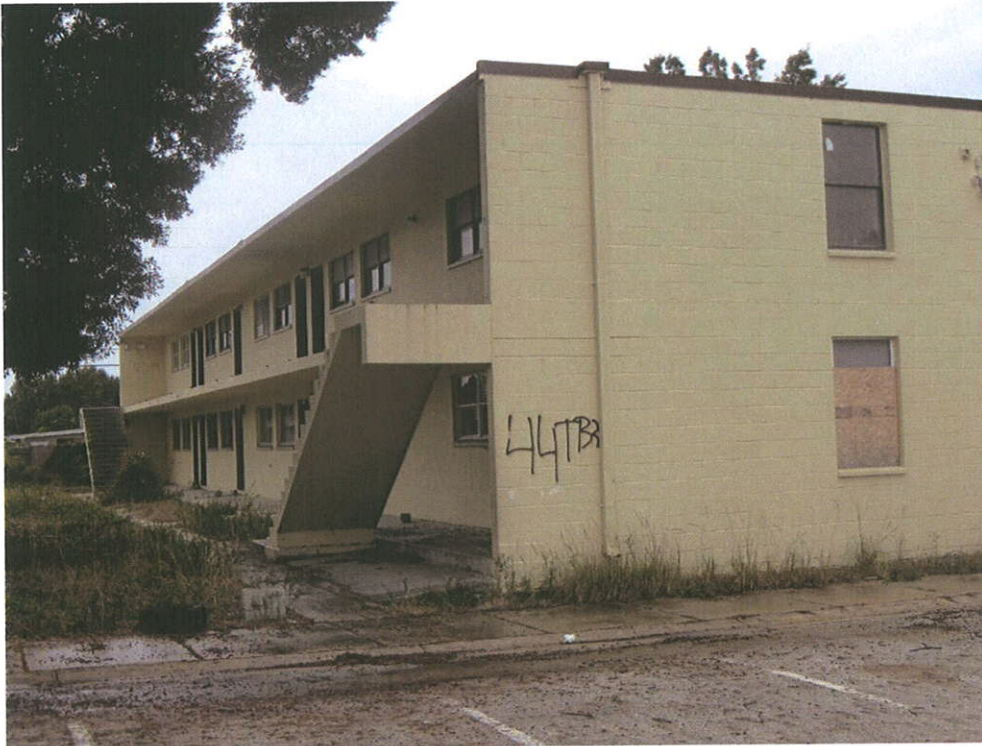
Photo 7: Gifford Gardens Apts. Building C front exterior
