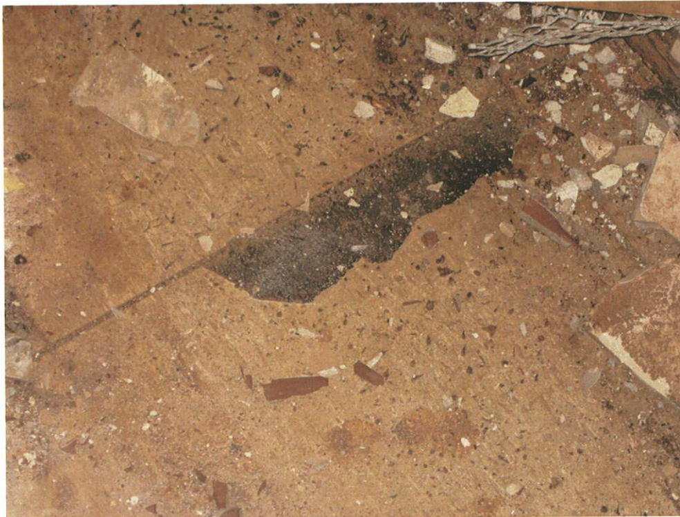
Photo 8: Typical ACM Tan VFT and black mastic in some units
