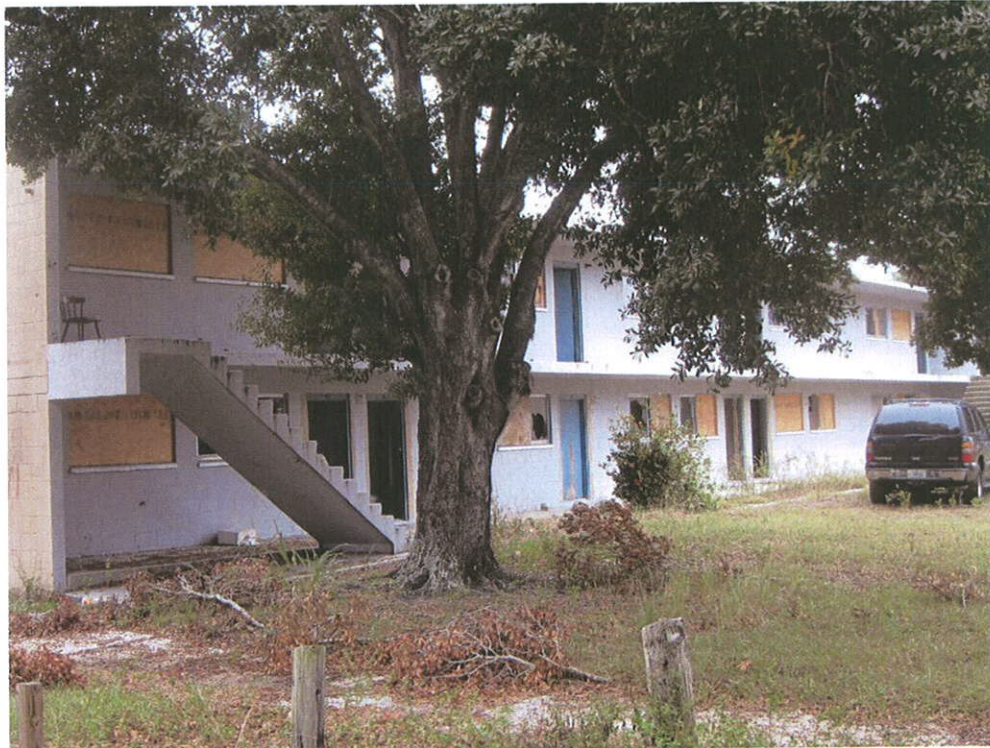
Photo 2: Gifford Gardens Apts. Building A front exterior
