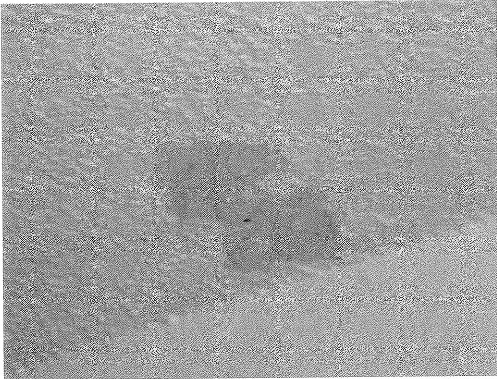
Photo 17: Typical ACM ceiling treatment (3%) in units
