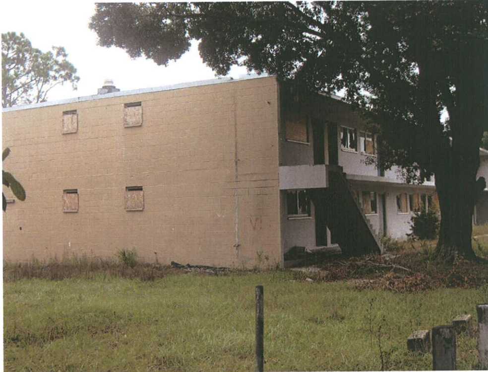
Photo 1: Gifford Gardens Apts. Building A rear exterior
