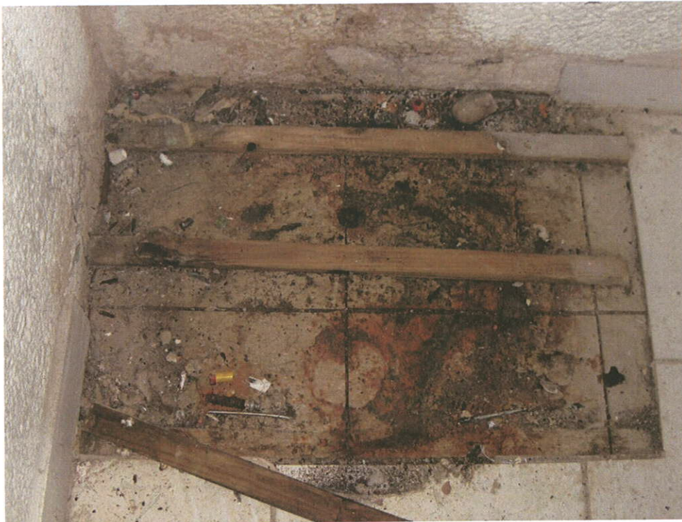
Photo 3: Typical ACM tan VFT under ceramic in water heater areas
