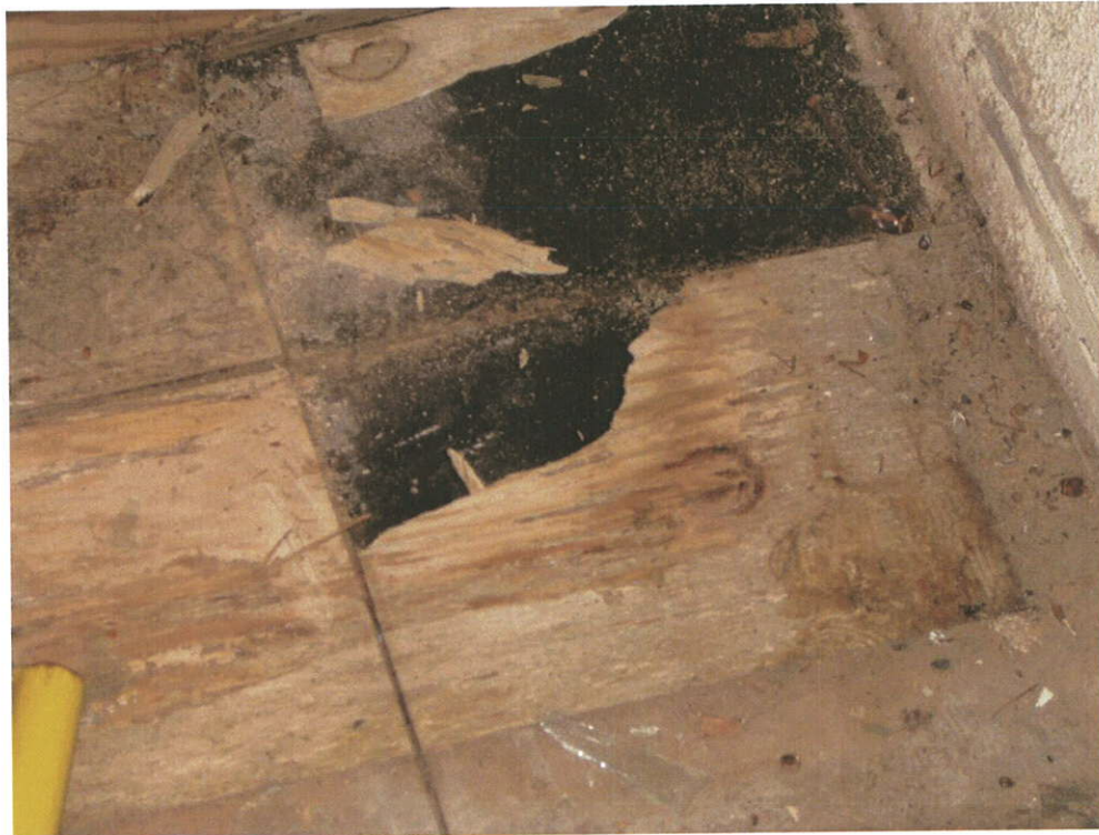
Photo 10: Typical ACM Tan VFT and black mastic in some units
